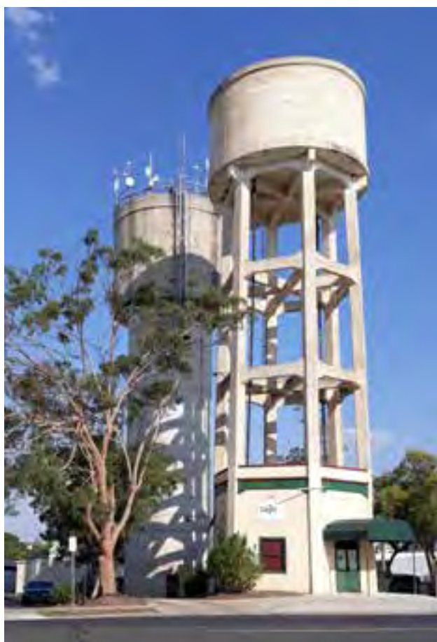
Water tower, Goondiwindi
