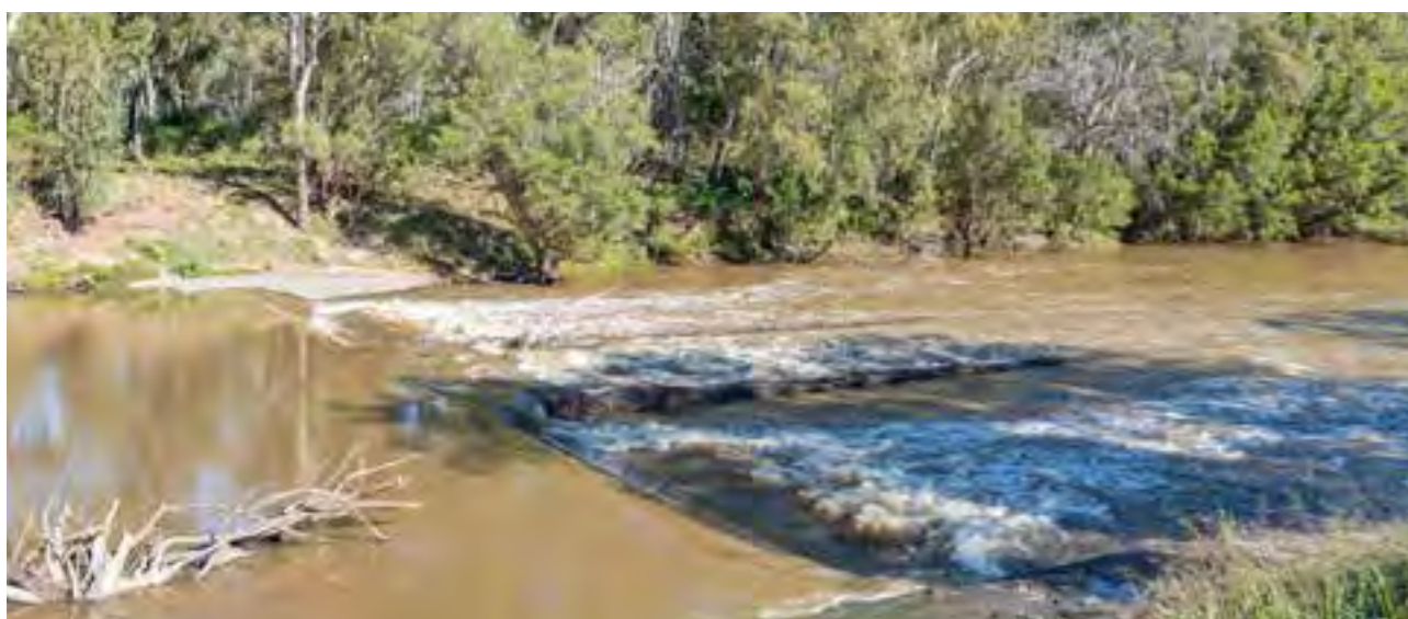
Paul Hilton weir, Goondiwindi
