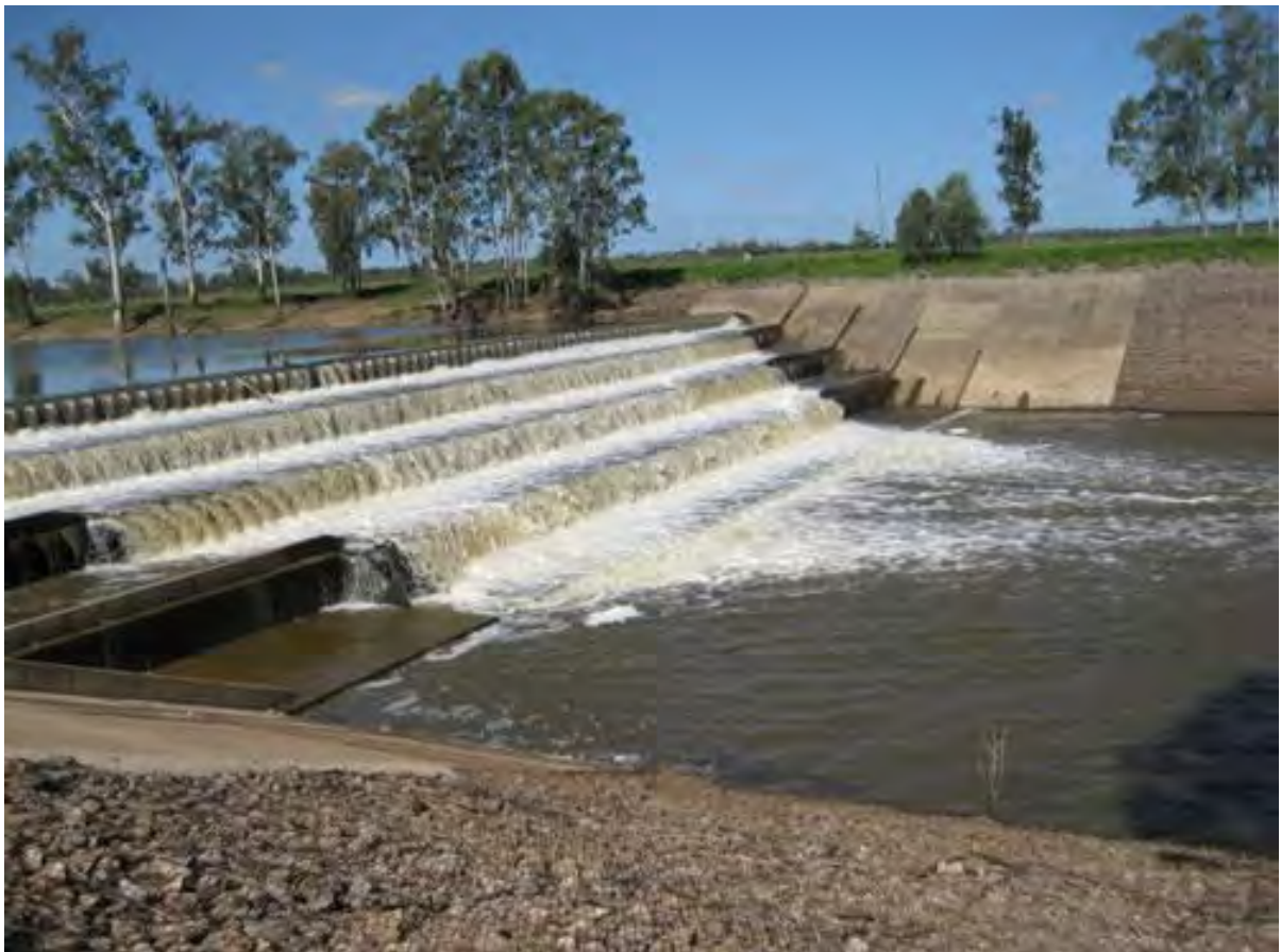
Figure 8 John Goleby Weir – Burnett River – Sheet piling weir
