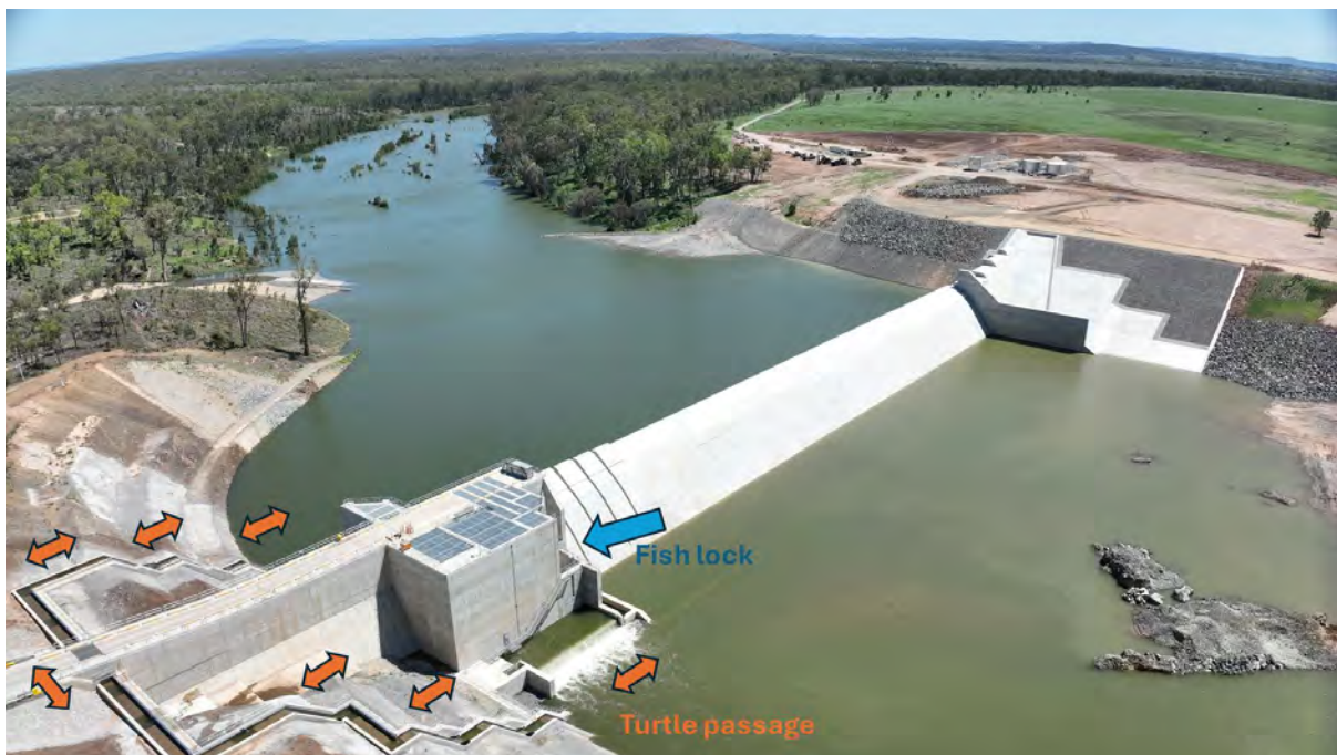
Figure 28 Turtle passage and fish lock at Rookwood Weir, Fitzroy River (Sunwater, 2025a)
