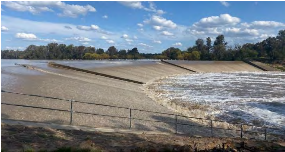
Figure 13 Lemontree Weir – Condamine River – minimum energy weir (Chanson, 2024)
