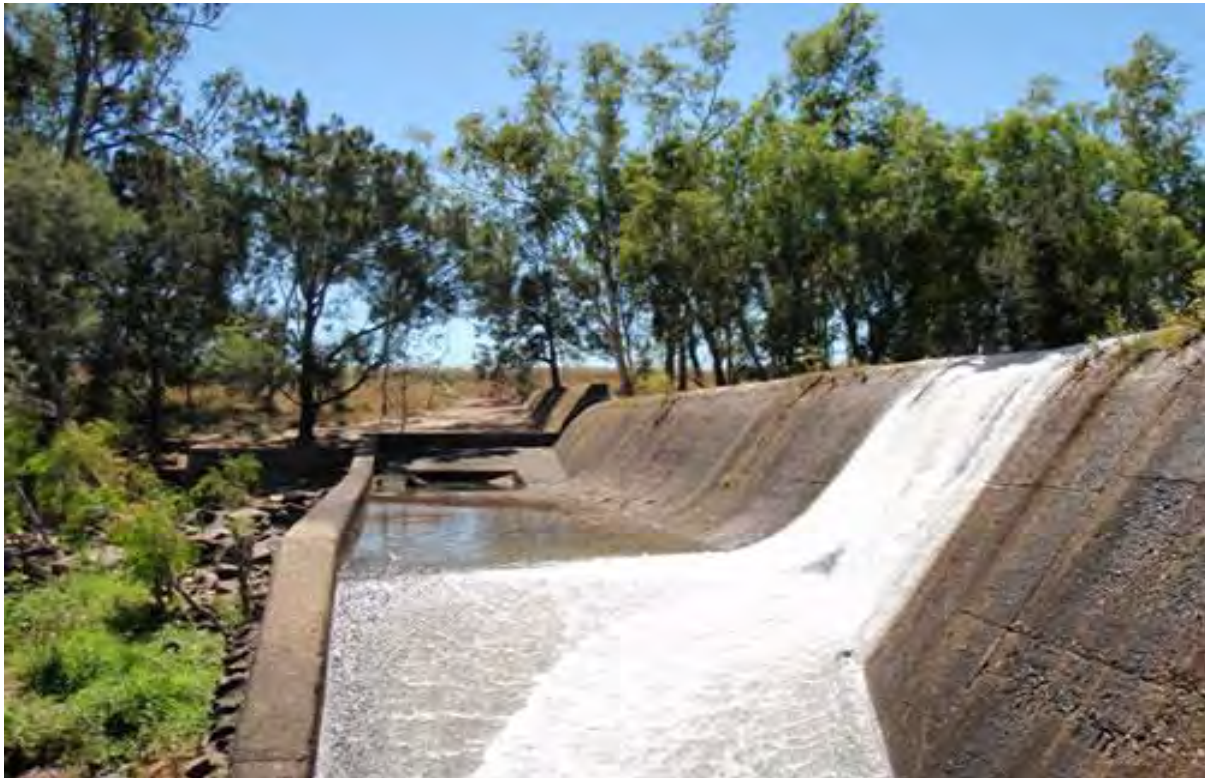
Figure 6 Leafgold Weir – Walsh River – concrete gravity
