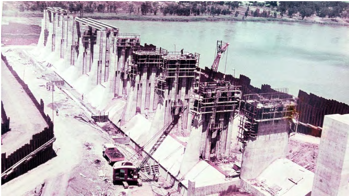
Figure 18 Fitzroy River Barrage during construction (RRC 2026)
