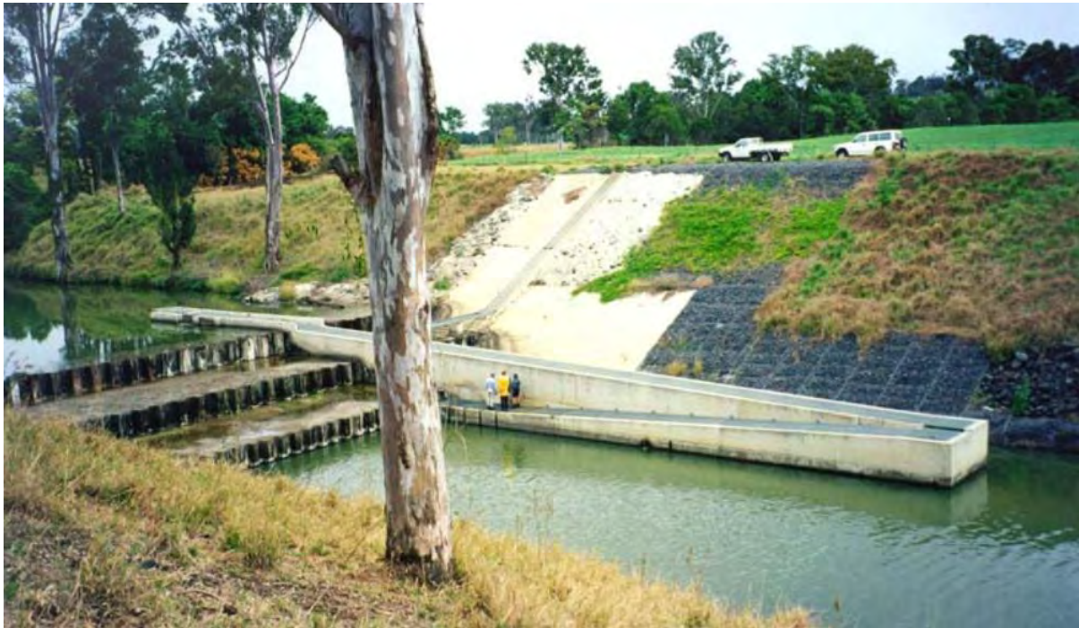
Figure 27 Fish lock at Eden Bann Weir, Fitzroy River (Sunwater, 2025)
