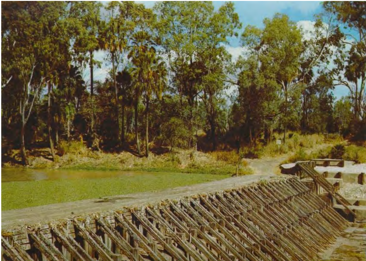
Figure 3 Theodore Weir – Dawson River – timber crib weir
