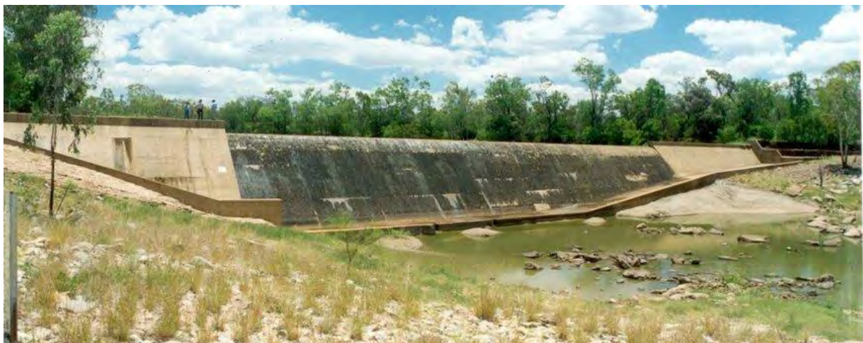
Figure 31 Neville Hewitt Weir - Dawson River – reconstructed top lift is clearly visible
