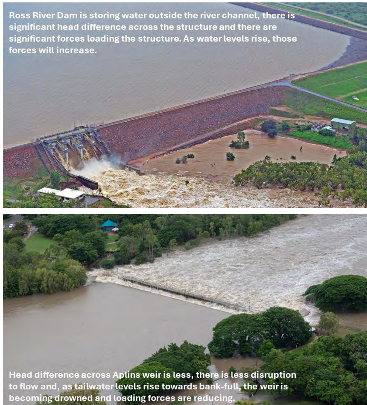
Figure 1 Ross River Dam (top) and Aplins Weir (bottom) during a flood event in 2019. Aplins Weir is approximately 20km downstream of Ross River Dam along the same watercourse.
