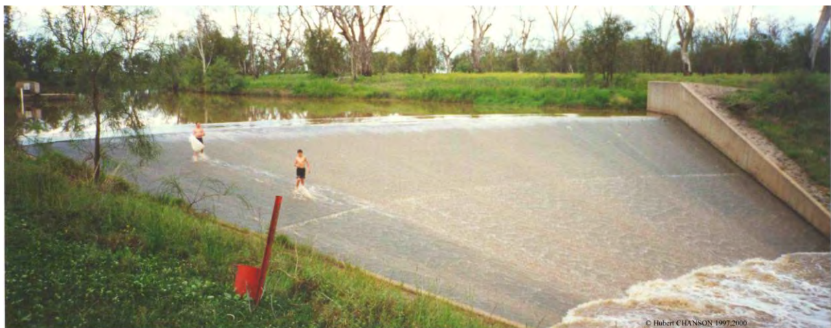
Figure 13 Lemontree Weir – Condamine River – minimum energy weir (Chanson, 2024)
