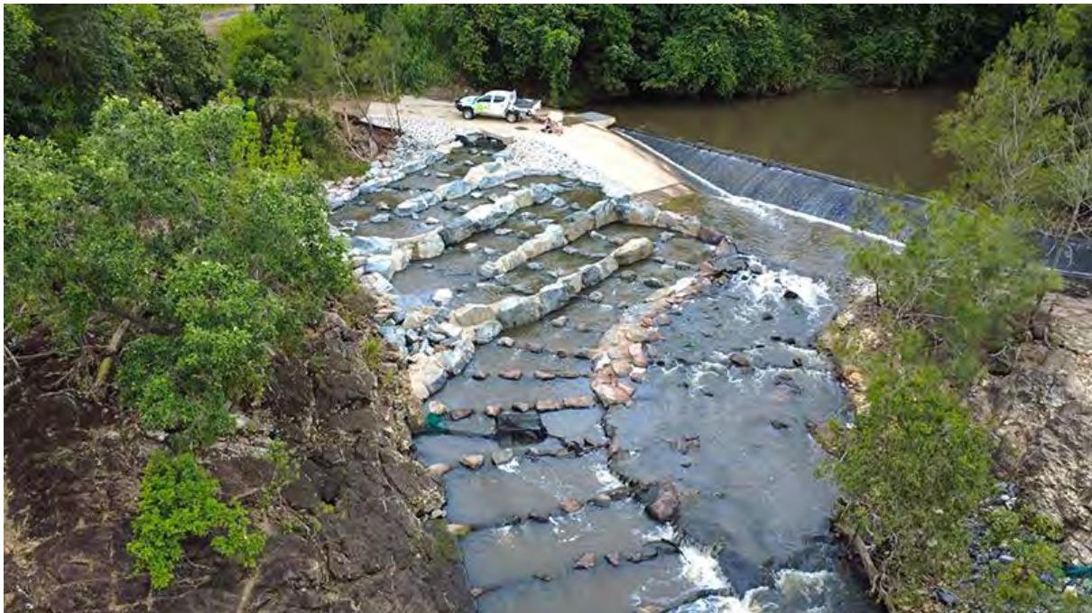
Figure 25 Rock ramp fishway at Jolimont Creek Weir (Catchment Solutions, 2025)
