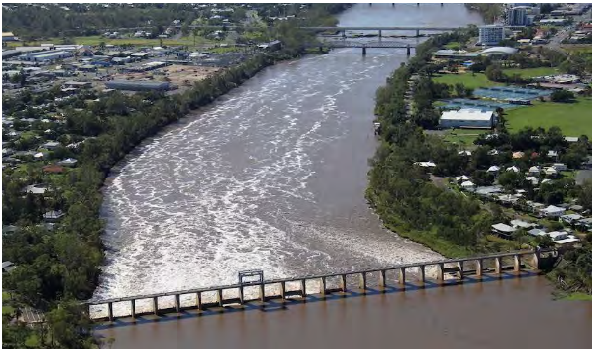
Figure 20 Fitzroy River Barrage during flood operation with several gates opened
