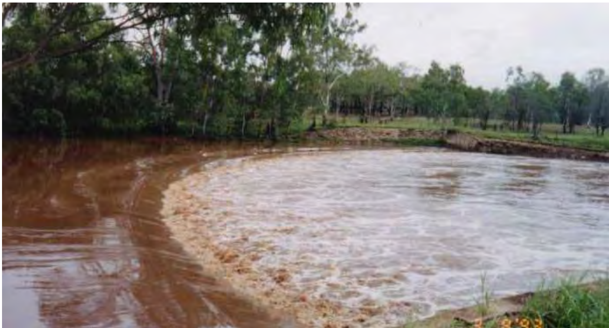
Figure 11 Clermont Weir – Sandy Creek - Minimum energy weir during flood overflow on 8 March 1993 (Chanson, 2024)
