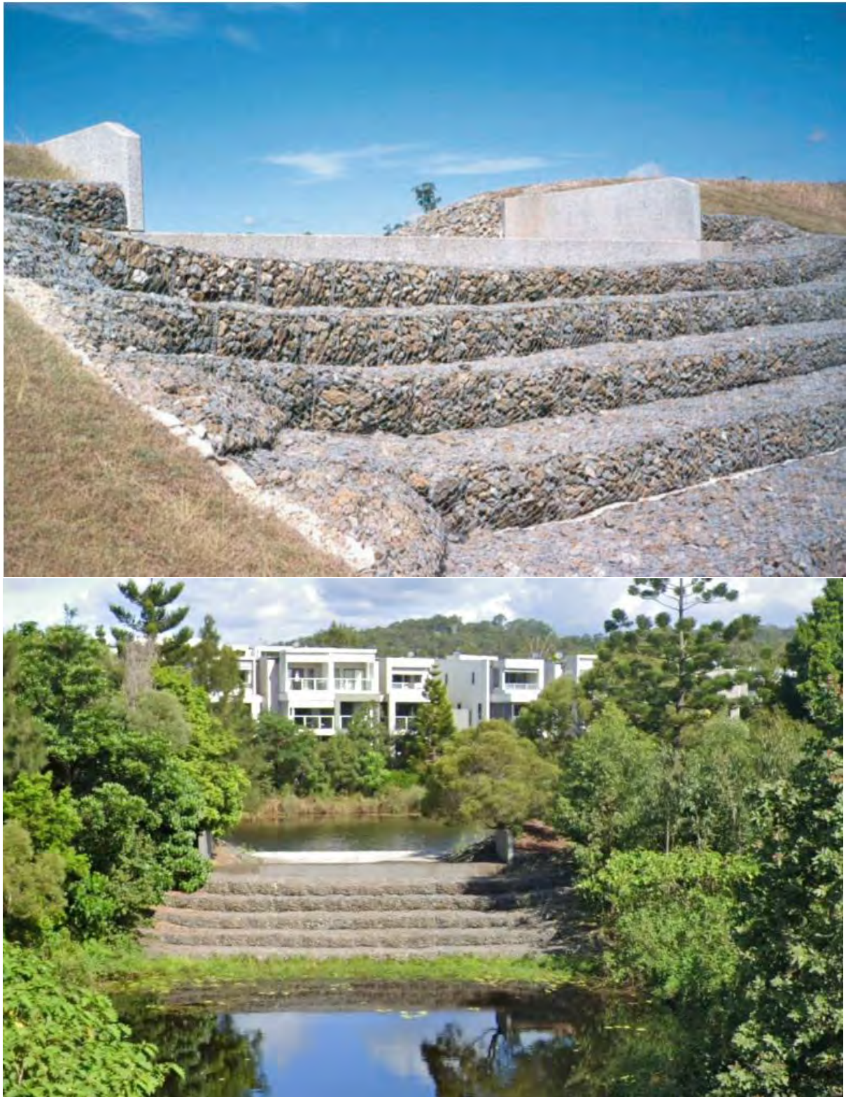
Figure 32 Gabion stepped weir at Robina, constructed in 1997 (top, Gonzalez et al 2008) and still operational (bottom, Google Maps). The weir impounds a small water body and is not exposed to high energy flow conditions.
