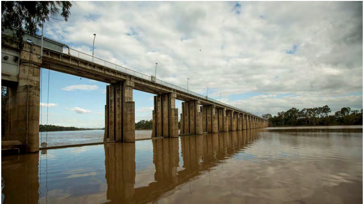
Figure 20 Fitzroy River Barrage during flood operation with several gates opened
