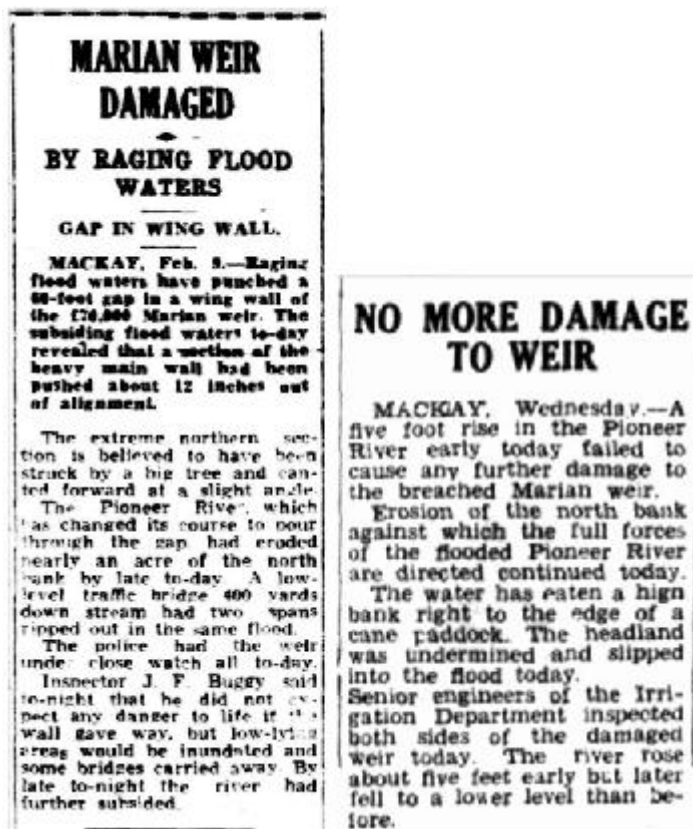
Figure 30 Newspaper articles describing the Marian Weir damage (Cairns Post, Wed 10 Feb 1954 and Bundaberg News, Thu 11 Feb 1954 (Trove, 2025))
