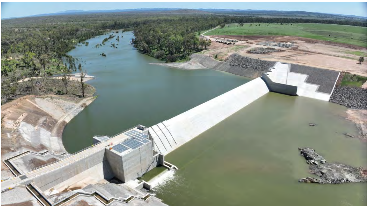
Figure 5 Rookwood Weir – Fitzroy River – concrete gravity
