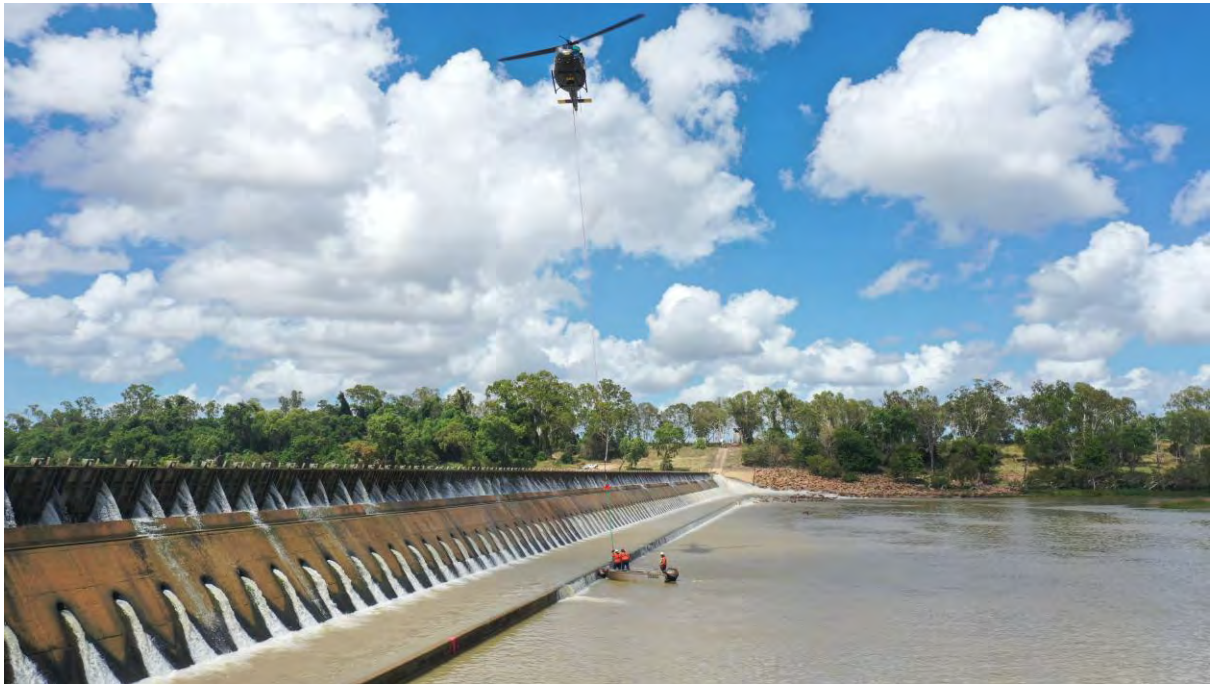
Figure 16 Ben Anderson Barrage – Burnett River – collapsible steel shutters (Sunwater 2021, Bundaberg Blasting 2020)
