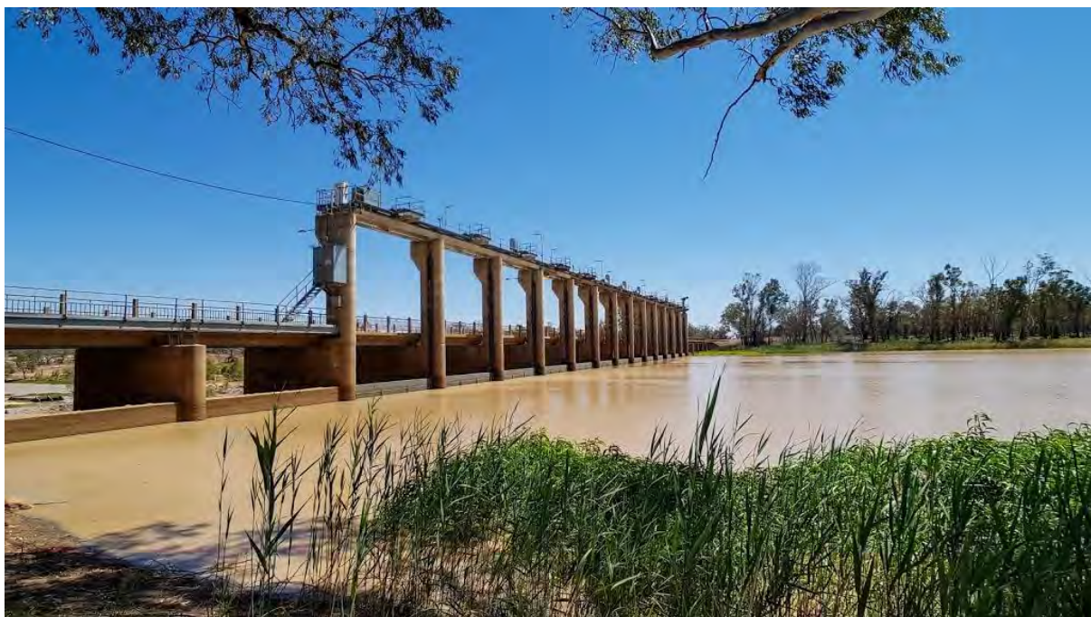
Figure 14 Jack Taylor Weir - Balonne River – vertical lift gates
