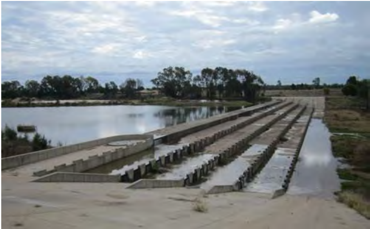
Figure 10 Moolabah Weir – Thuraggi watercourse – damage occurred to the spillway, with movement of concrete slabs, during flooding in 2012
