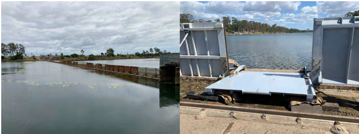
Figure 16 Ben Anderson Barrage – Burnett River – collapsible steel shutters (Sunwater 2021, Bundaberg Blasting 2020)
